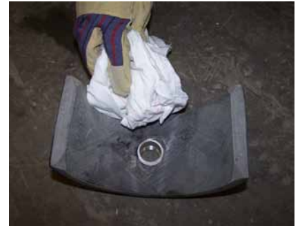
Wipe the sanded saddle and pipe surfaces clean
