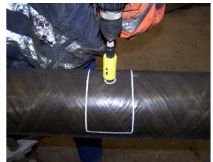
When required mark and drill the hole opening
