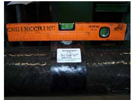
Push saddle into place and check the alignment
