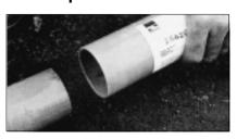
The spigot end should be inserted without rotation until contact of the matching taper in the bell is felt. At this point, the loose joint component should be slightly rotated while applying force to the joint. A small reverse twist will "lock" the joint. This rotation of the joint end will redistribute the adhesive evenly and work any air out of the bond line.
