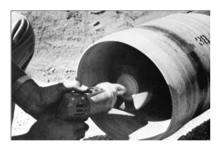
Remove the exterior gloss up to the recorded insertion depth using a flapper sander or sandpaper. A light sanding of the spigot (if factory made) should also be done.
