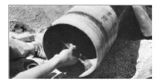
Apply properly mixed adhesive to both the bell and spigot bonding surfaces.
